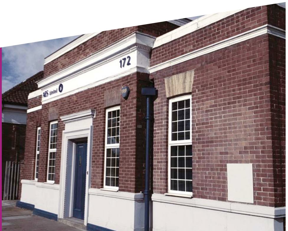
Headquarters of AES Digital Solutions in Billingham
