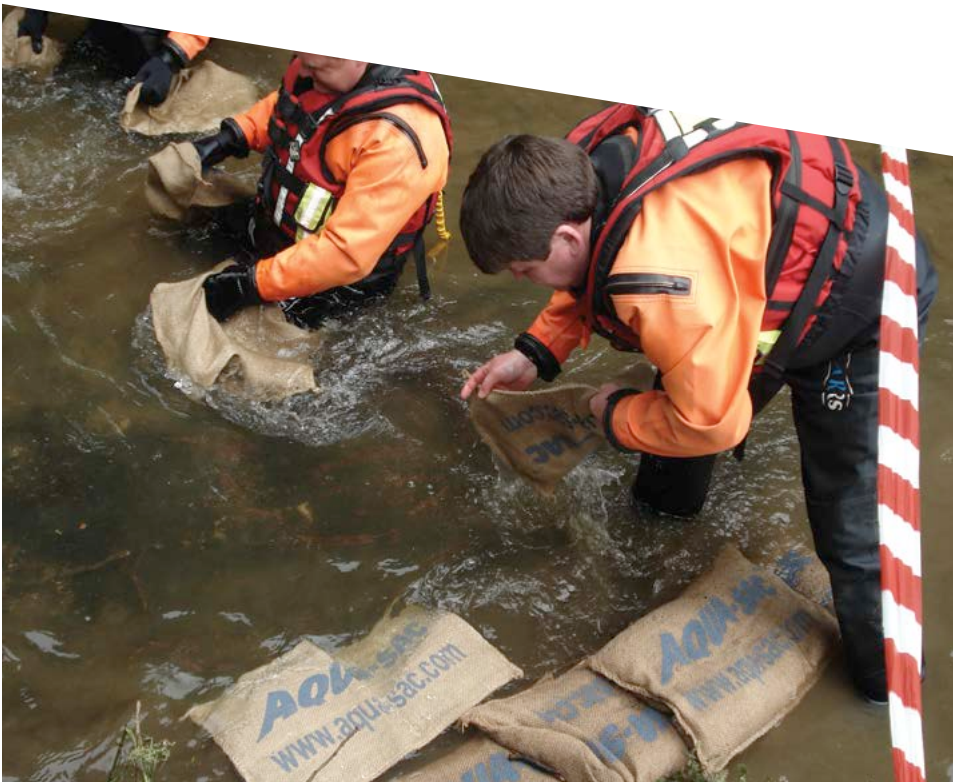
AET Flood Defence's main product, Aqua-Sac®, at work
