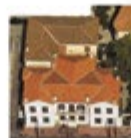
Athens, Building A
